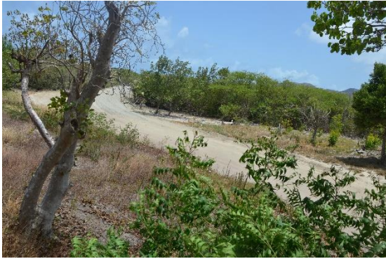
Central Access Road (looking landward)
