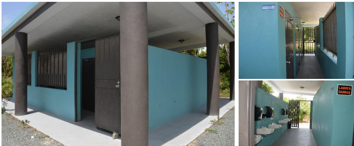
Figure 2-22. Public restroom facility near the central entrance at Long Bay, Beef Island
