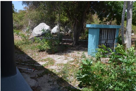
View of water meter
