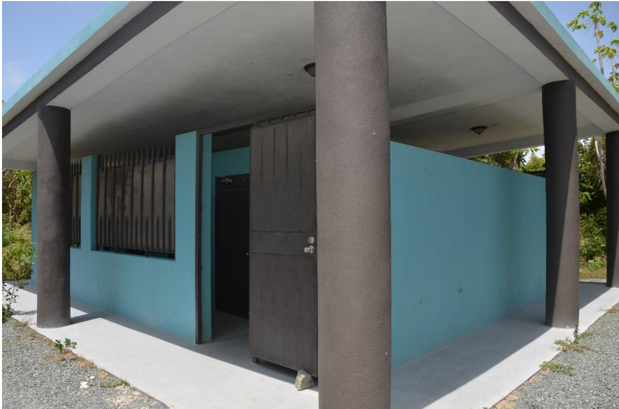
Figure 6-41. Existing public restroom facility The entrance into the male stalls is shown. The entrance to the female stalls is on the opposite side.
